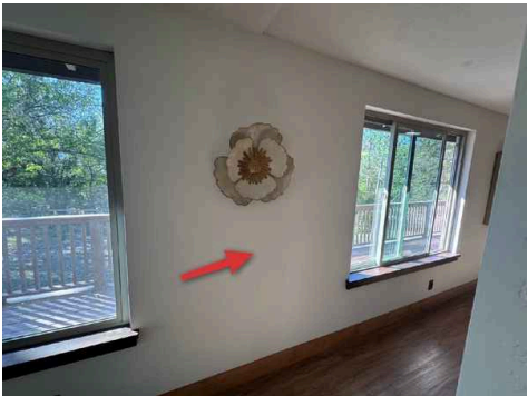
Dining Room to Kitchen Wall
