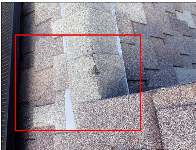
1.0 ROOF COVERING (Picture 1)
