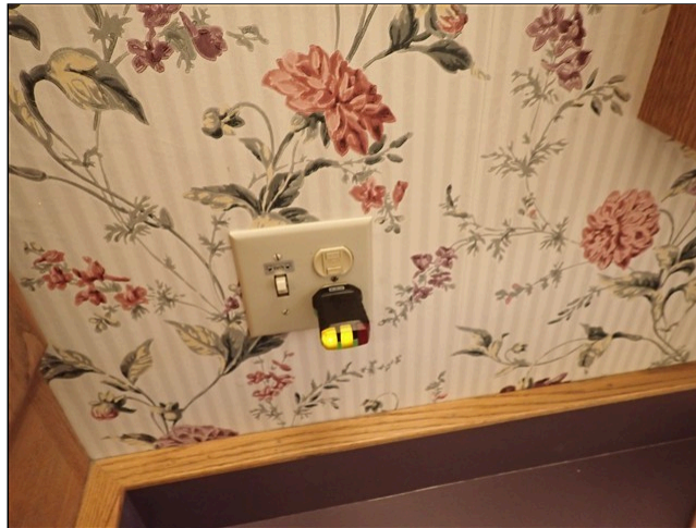
7.6.C ELECTRIC / GFCI (Picture 1)
