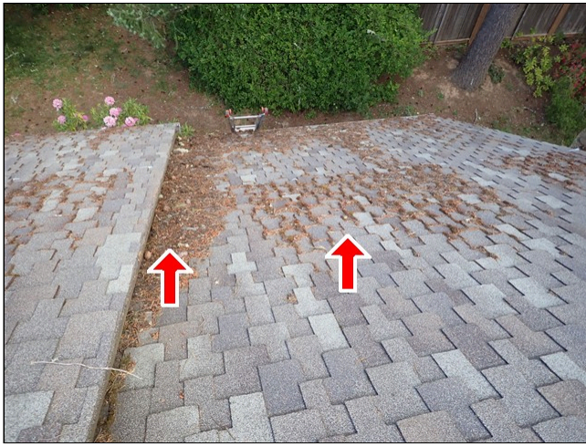
1.0 ROOF COVERING (Picture 3)
