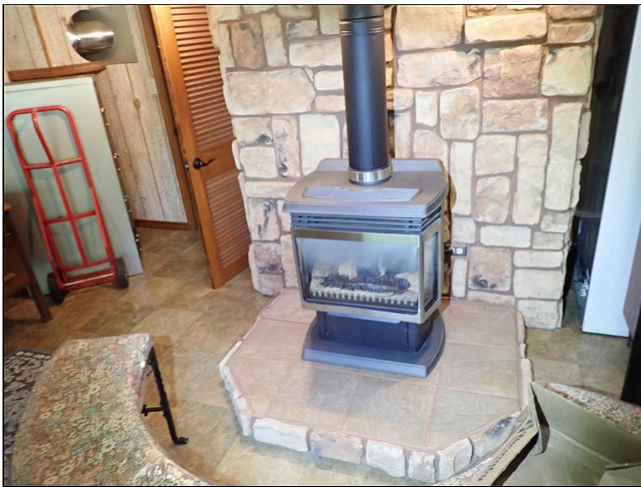
5.9 FIREPLACE (BASEMENT) (Picture 1)
