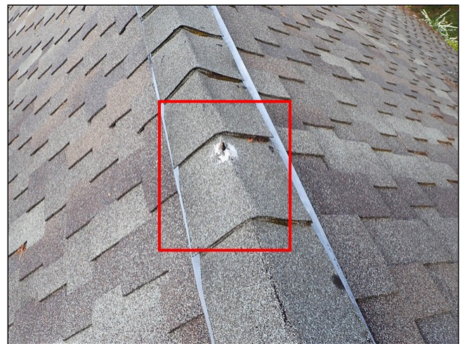
1.0 ROOF COVERING (Picture 2)
