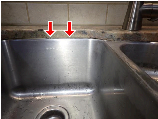
7.0 PLUMBING / SINK (Picture 1)
