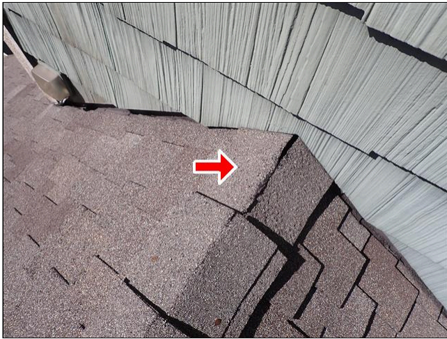
1.0 ROOF COVERING (Picture 5)
