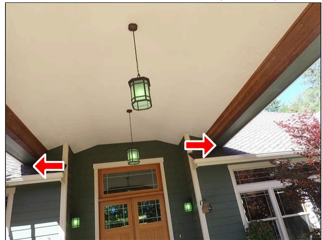
1.6(2) RAIN GUTTERS (Picture 1)
