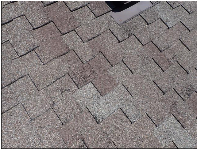
1.0 ROOF COVERING (Picture 1)
