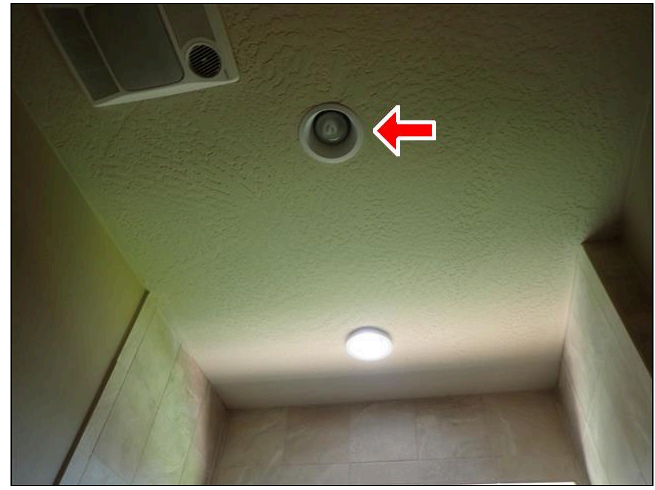
11.5 DEVICES (Picture 1) Hallway Bath
