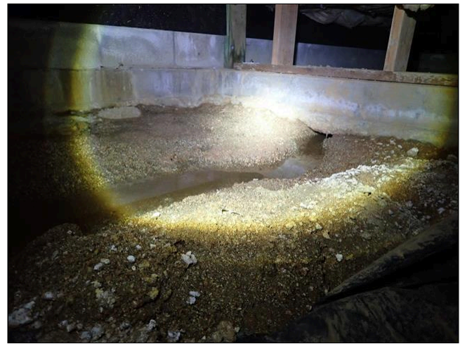
10.0 EXTERIOR FEATURES / WATER INTRUSION FACTORS (Picture 4) Right Section
