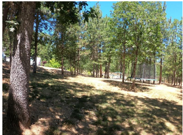
View of Drain Field (tank to left)
