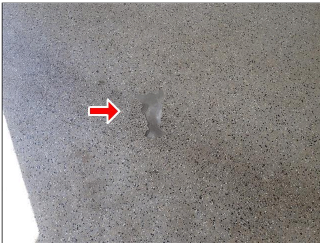
4.0 FLOOR SLAB (Picture 1)
