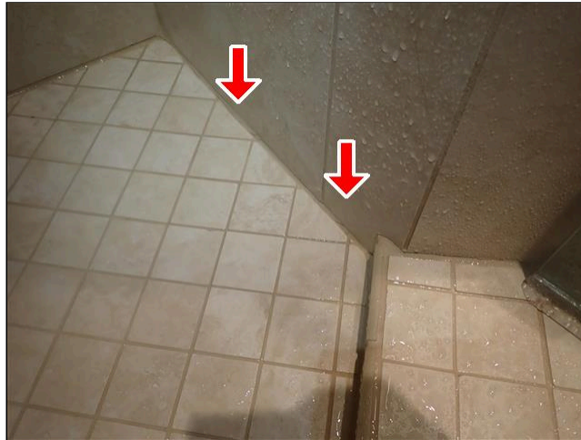
8.3.B SURROUND / ENCLOSURE (Picture 1)
