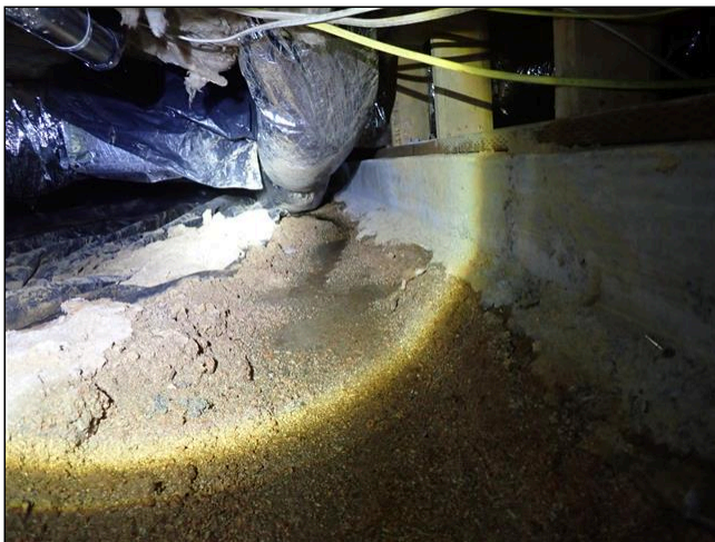
9.2 CRAWLSPACE FLOOR (Picture 1)
