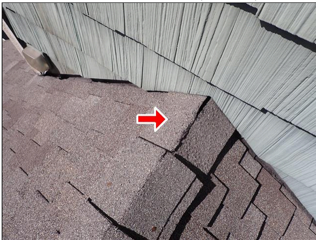
1.0 ROOF COVERING (Picture 5)
