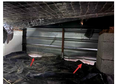
Back Of Home Under Deck
