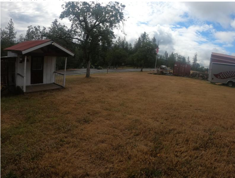
View of Drain Field from end of Sand Filter
