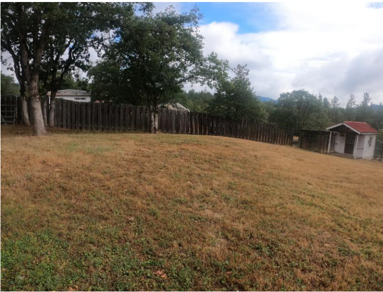
View of Sand Filter from Tank
