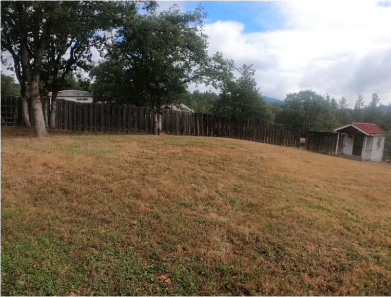
View of Sand Filter from Tank
