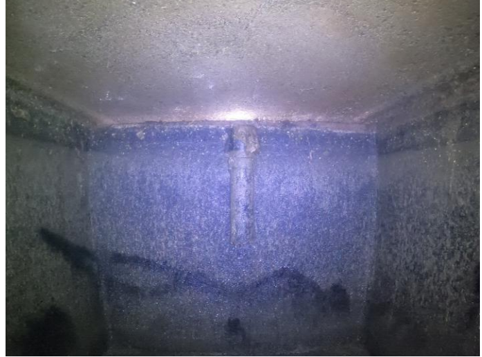
Interior Outlet Baffle
