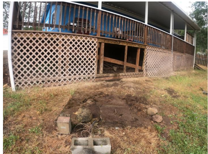
View of Lids to House
