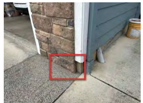
Front Right Of Home
