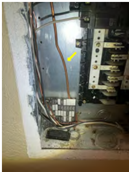
Panel B copper ground wire
