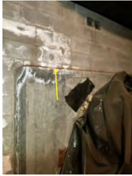
small amount of efflorescence in the crawlspace normal for age of home
