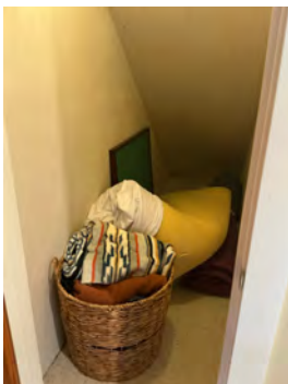
Under the stairs in basement closet
