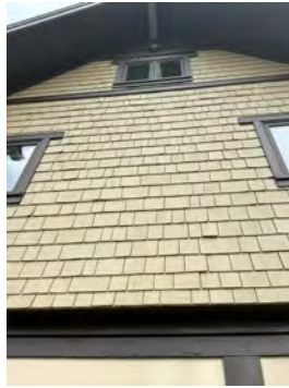
siding on the home looks in good shape
