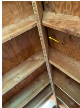
ridge vent in attic space
