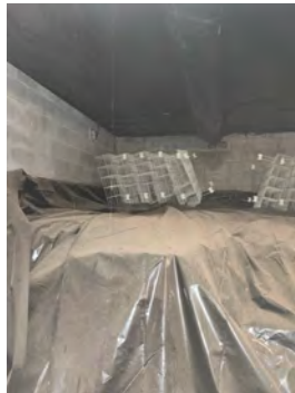
Vapor barrier good in the crawlspace
