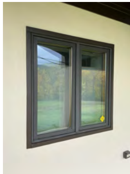
Window trim in good shape on the home
