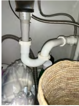
No sign of leaking under laundry bathroom sink at this time
