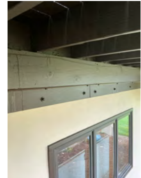
Steel L iron supporting ledger board on decks, very good and strong
