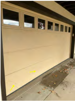
Damaged bottom panel of the garage door, recommend lic contractor replace bottom panel
