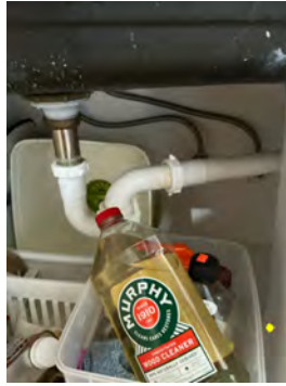
No sign of leaking under laundry sink at this time
