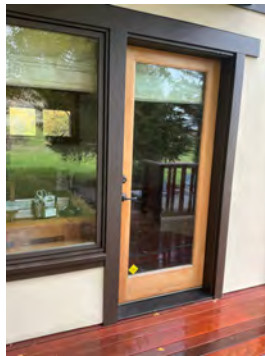
North office door
