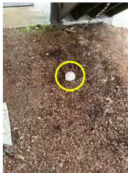
Sewer clean out on West side of home under deck stairs
