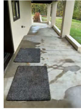
West patio under deck
