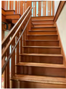
stairs in good shape handrail nice and solid
