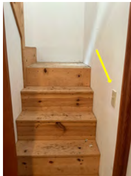
No handrail going up to storage area in attic space
