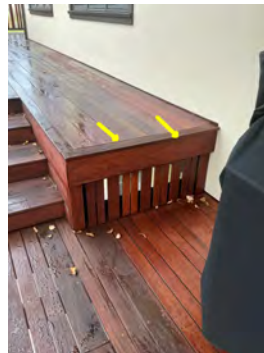
possible fall hazard on west end of the deck, recommend scooting BBQ closer or installing handrail
