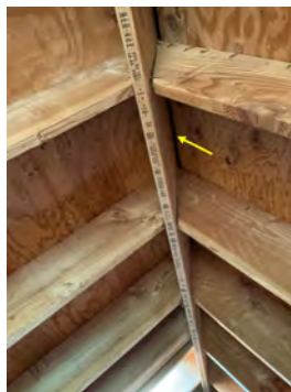
ridge vent in attic space
