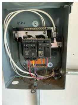
Garage sub panel in good shape
