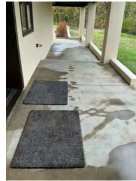
West patio under deck
