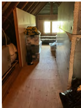
storage space in attic
