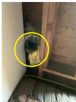
North end of attic bath fan vented into attic, recommend this be vented to the exterior
