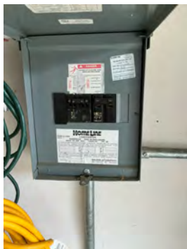
Garage sub panel in good shape
