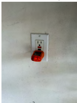
Garage GFCI works good
