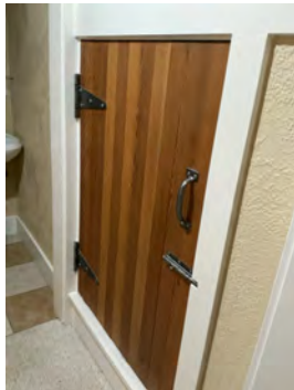
Crawlspace door in the basement
