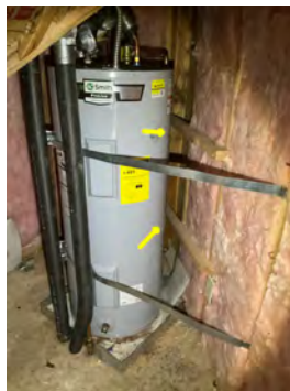
need blocks behind water heater to make unit solid so does not move in a earthquake
