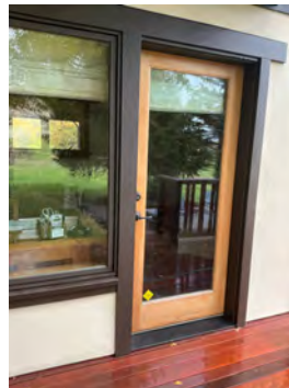
North office door
