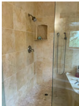
Handles and nozzle loose in master tub, recommend a lic plumber secure these properly
