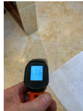
Radiant heating working in master bath.
