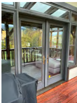
West living room doors
