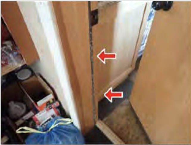
4.6 HOUSE / SERVICE DOOR (Picture 2)
