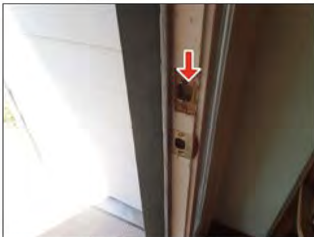
2.3 ENTRY DOORS (Picture 1)
