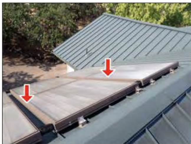
1.0 ROOF COVERING (Picture 3)
