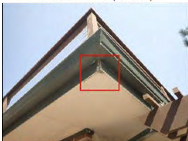
1.5 FASCIA / SOFFITS (Picture 2)
