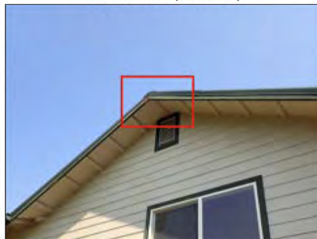
1.5 FASCIA / SOFFITS (Picture 1)
