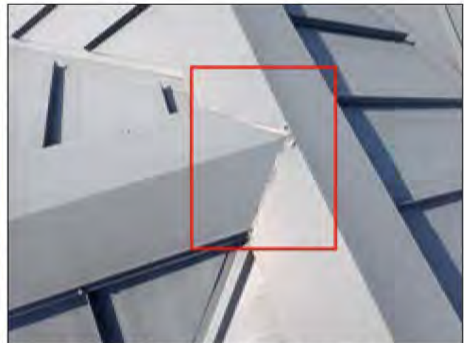
1.0 ROOF COVERING (Picture 2)
