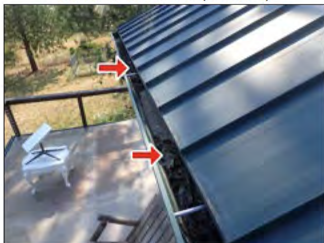
1.3 RAIN GUTTERS (Picture 1)
