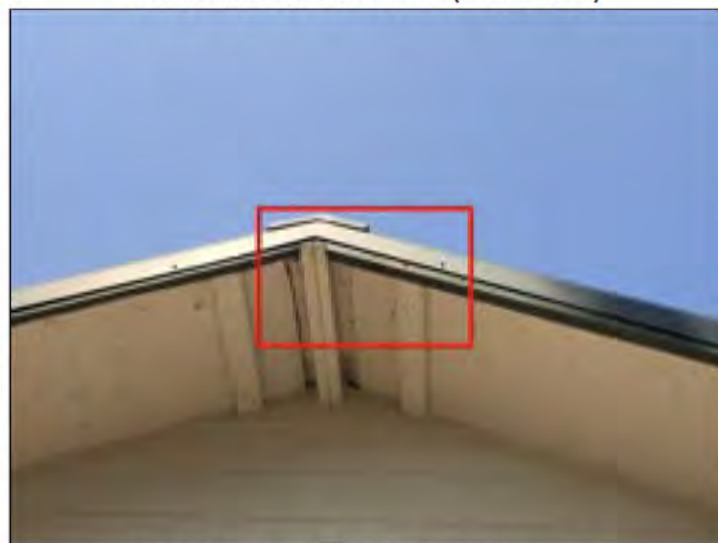
1.5 FASCIA / SOFFITS (Picture 3)
