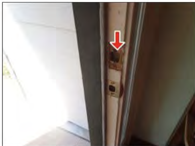
2.3 ENTRY DOORS (Picture 1)
