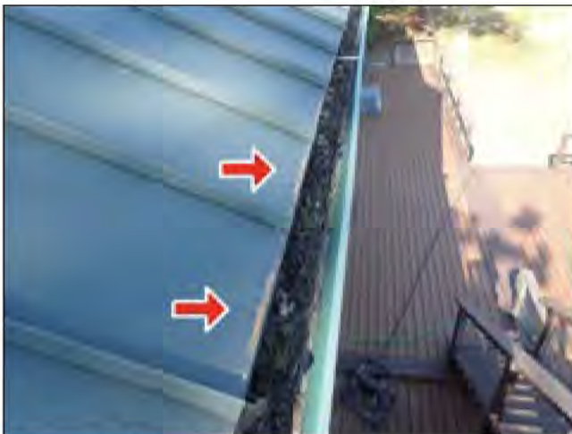
1.0 ROOF COVERING (Picture 1)
