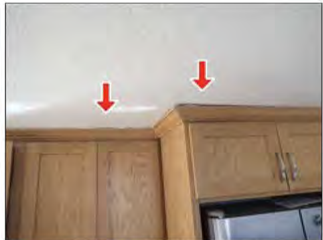
7.1 WALLS / CEILING (Picture 1)
