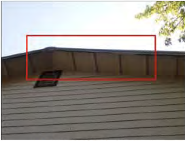
1.5 FASCIA / SOFFITS (Picture 4)
