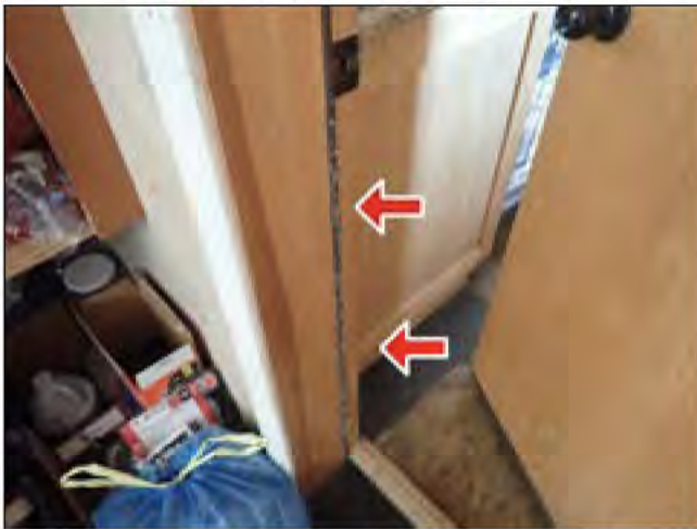
4.6 HOUSE / SERVICE DOOR (Picture 2)
