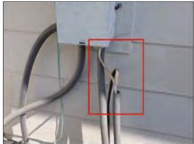
10.7 WIRING / CONDUCTORS (Picture 1)
