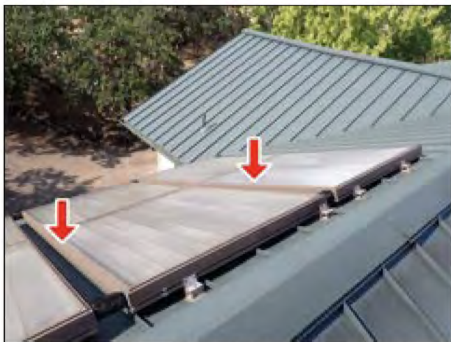
1.0 ROOF COVERING (Picture 3)
