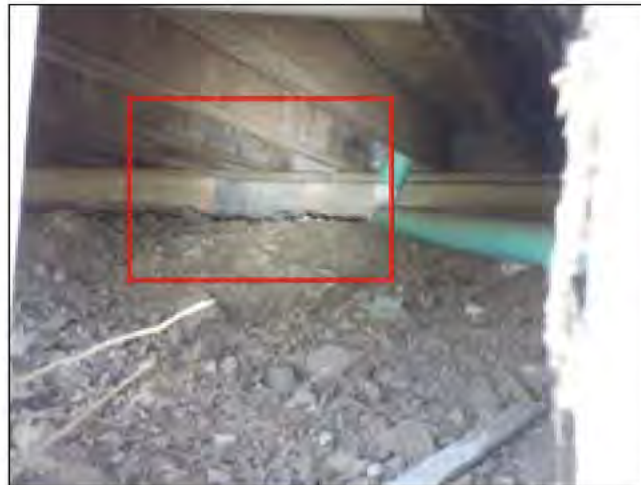
9.0 SLAB EXTERIOR / EDGE (Picture 1)
