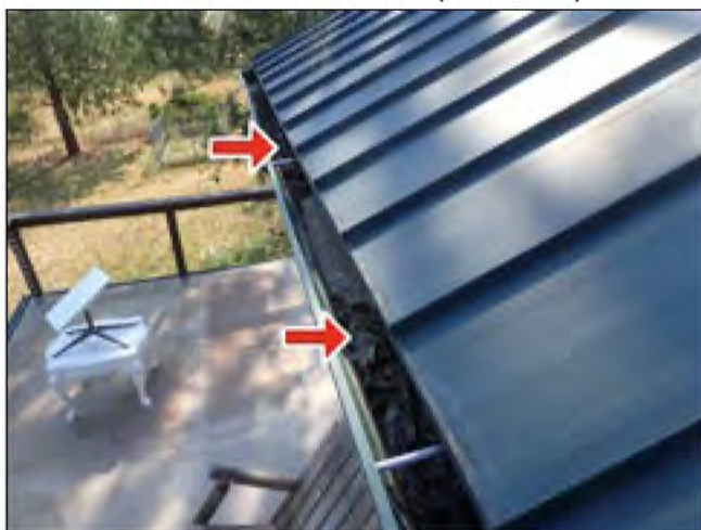
1.3 RAIN GUTTERS (Picture 1)
