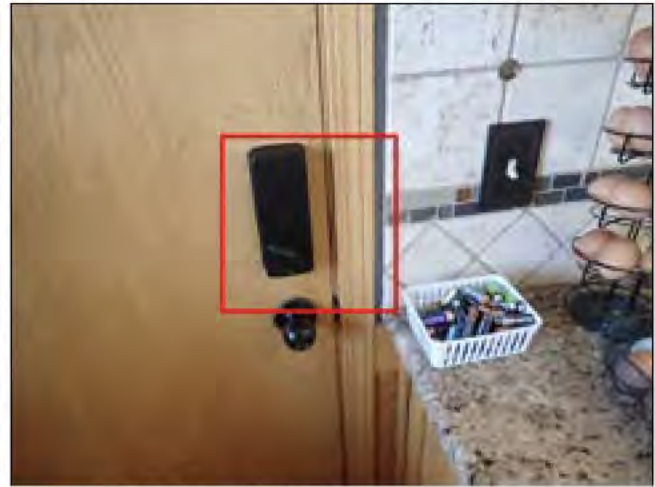
4.6 HOUSE / SERVICE DOOR (Picture 1)
