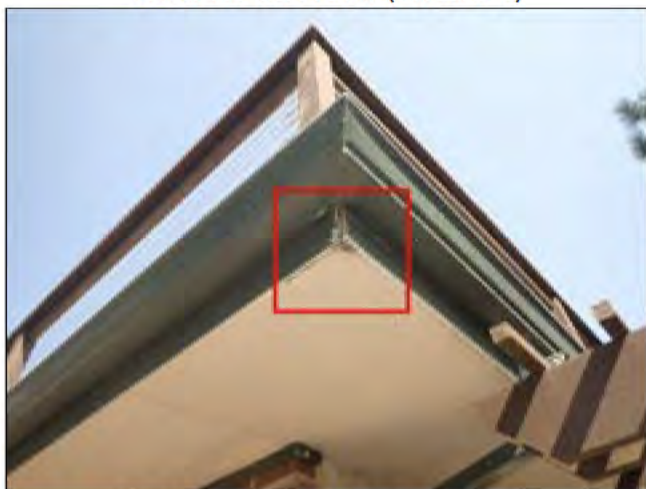
1.5 FASCIA / SOFFITS (Picture 2)
