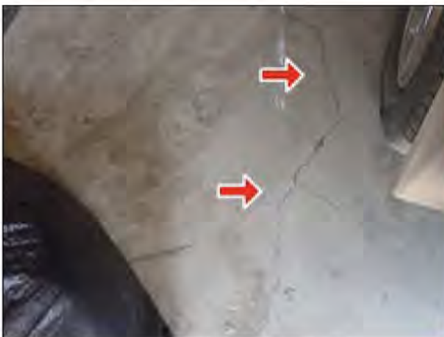
4.1 FLOOR SLAB (Picture 1)
