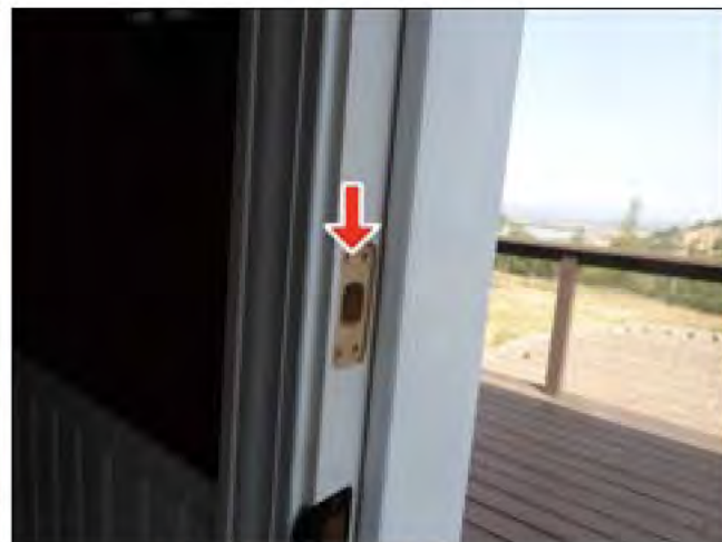
2.3 ENTRY DOORS (Picture 2)
