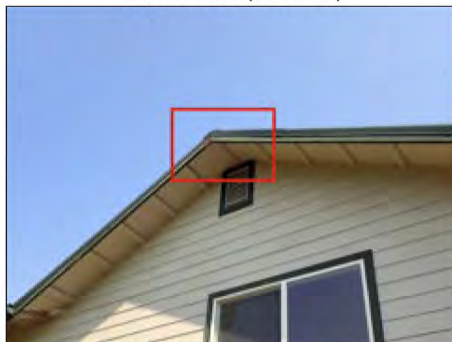
1.5 FASCIA / SOFFITS (Picture 1)
