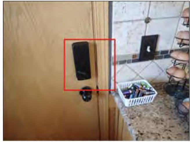
4.6 HOUSE / SERVICE DOOR (Picture 1)
