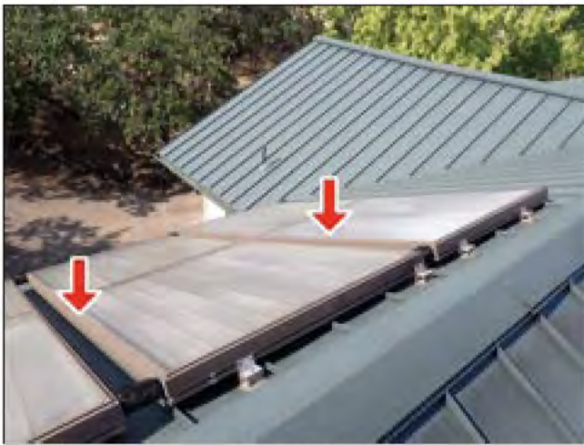
1.0 ROOF COVERING (Picture 3)
