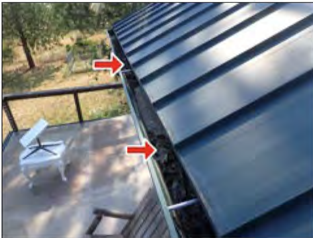
1.3 RAIN GUTTERS (Picture 1)
