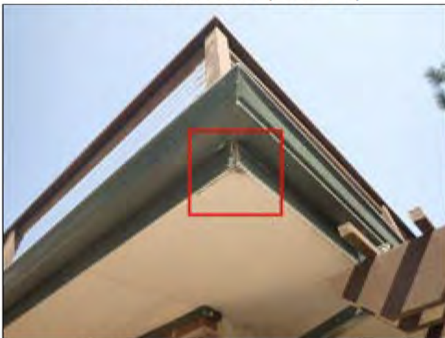
1.5 FASCIA / SOFFITS (Picture 2)
