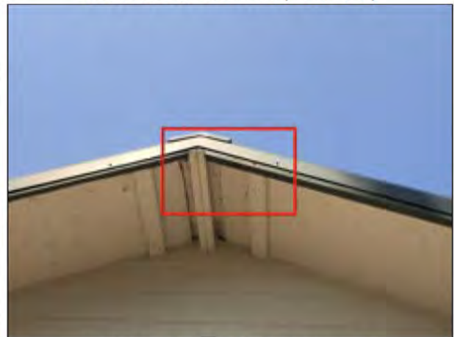
1.5 FASCIA / SOFFITS (Picture 3)
