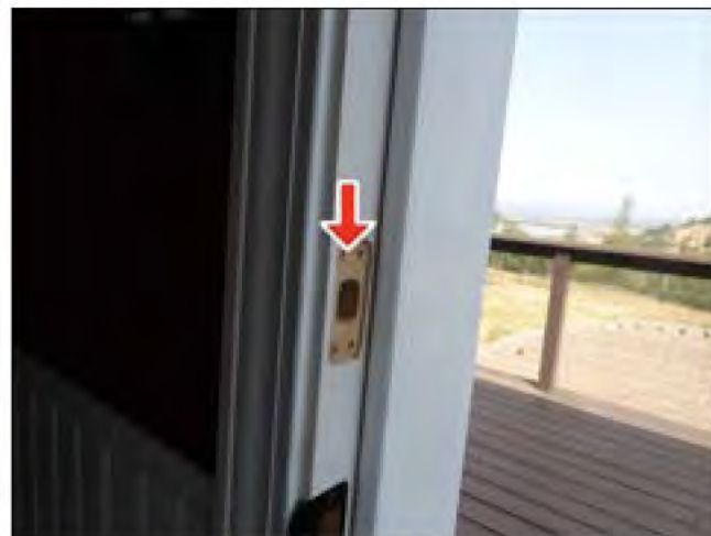
2.3 ENTRY DOORS (Picture 2)
