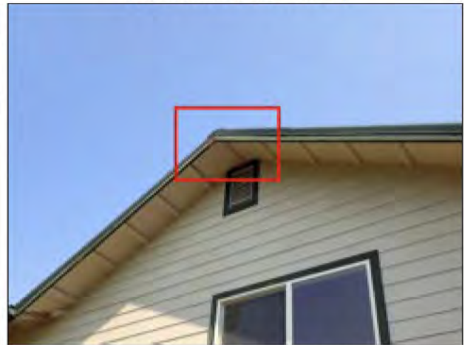
1.5 FASCIA / SOFFITS (Picture 1)
