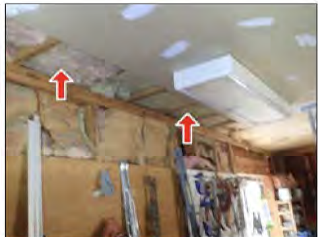
4.2 WALLS / CEILINGS (Picture 1)
