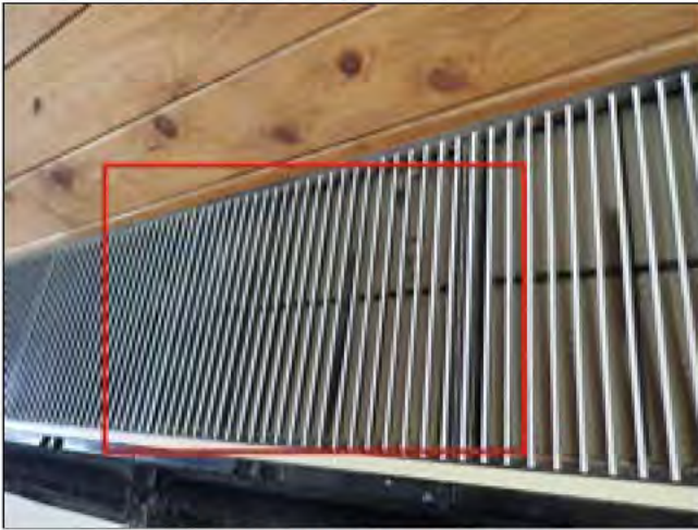
11.5 AIR HANDLER (Picture 1)
