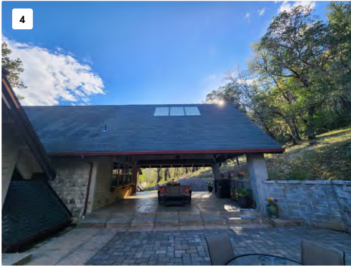
Project: 3998 Little Applegate Rd Date: Apr 6, 2026, 9:15 AM Creator: Dan Daulton
