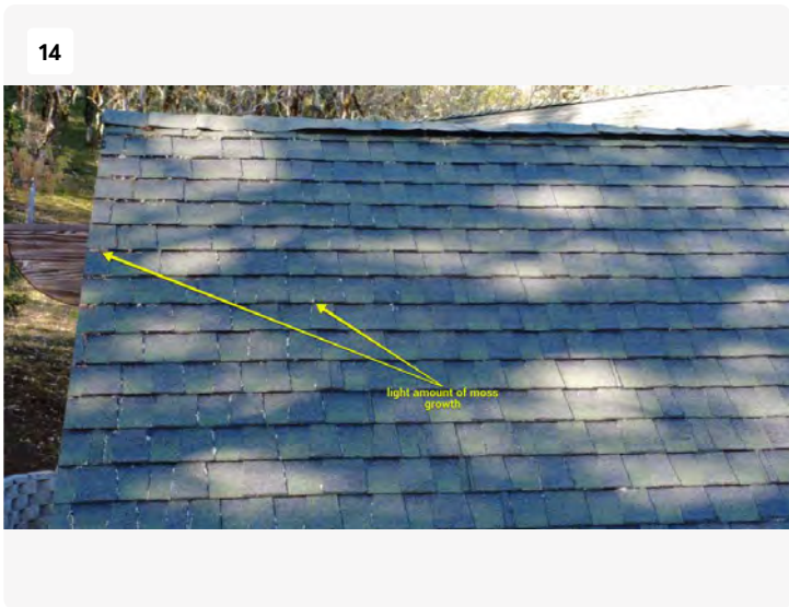
at a glance it looks like the edges of the dimensional portion of the shingles are worn and showing fiberglass, but once you zoom in the pictures you can see that it is light moss growth.
