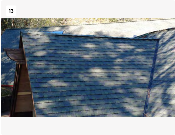
Project: 3998 Little Applegate Rd Date: Apr 6, 2026, 9:23 AM Creator: Dan Daulton
