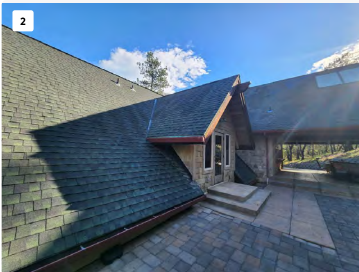
Project: 3998 Little Applegate Rd Date: Apr 6, 2026, 9:14 AM Creator: Dan Daulton
