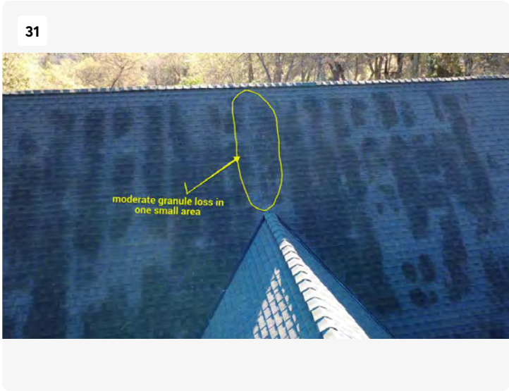
Project: 3998 Little Applegate Rd Date: Apr 6, 2026, 9:36 AM Creator: Dan Daulton
