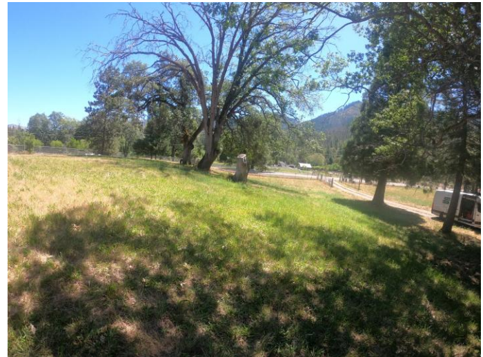
View of Drain Field from Tank
